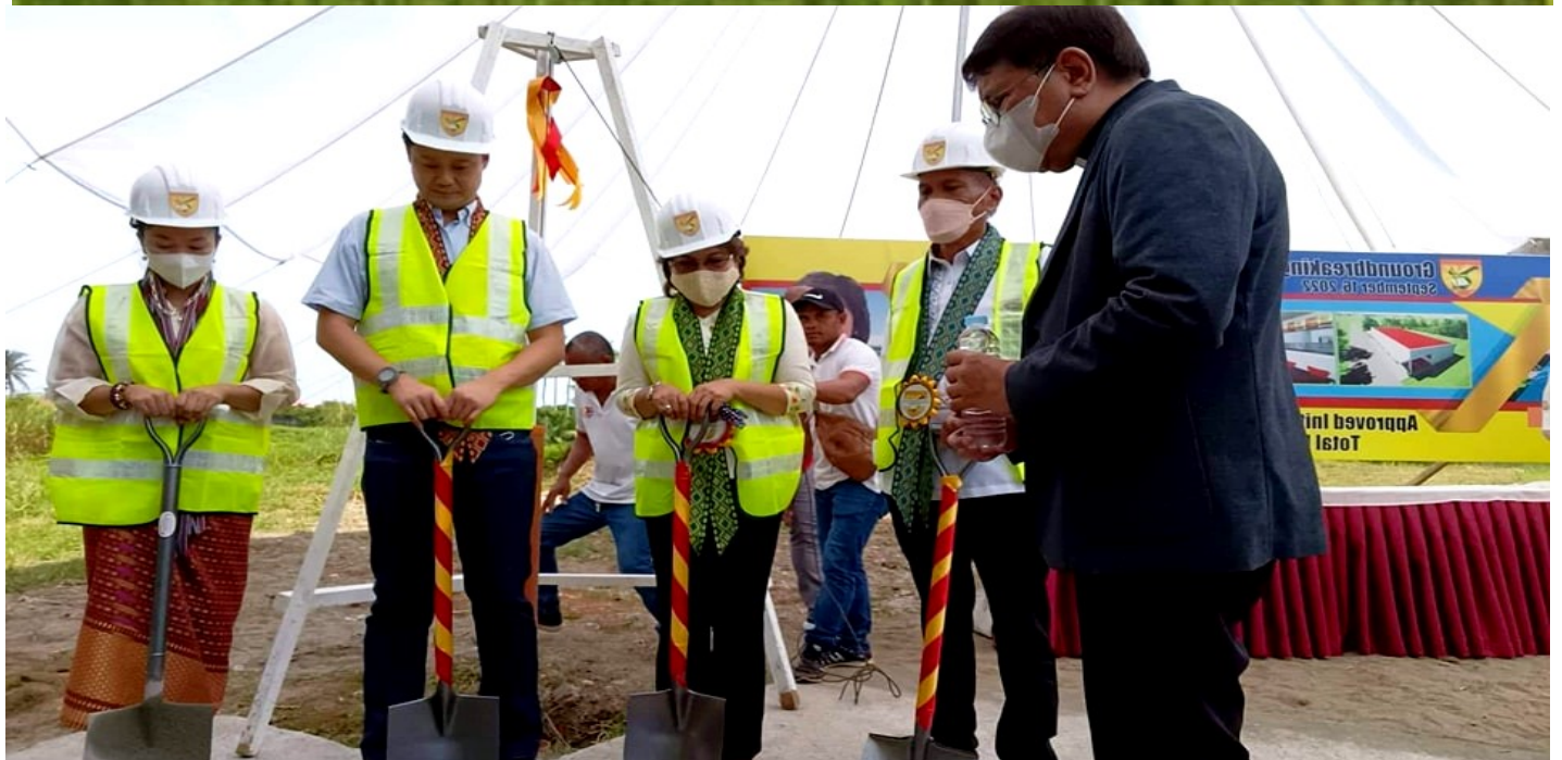
Site Blessing. Rev. Fr. Ranhilio C. Aquino, SJD officiates the blessing of the construction site of the new CSUA Food Court.
